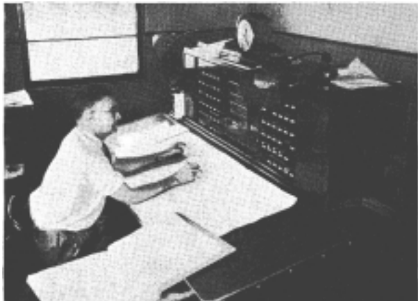
Figure 1 - Train Control Desk in Sydney, 1948
