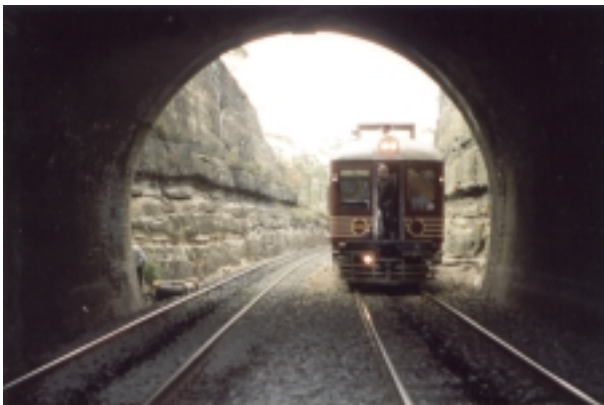
Figure 5 : Tunnel coverage survey for train radio
