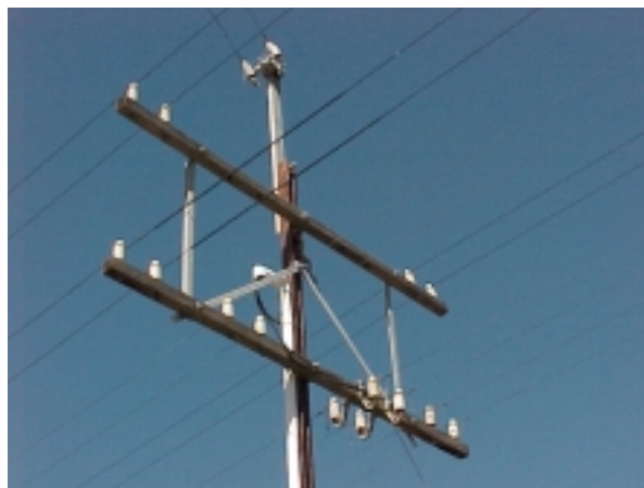
Figure 2: Toodyay – Kalgoorlie Steel Pole 6
