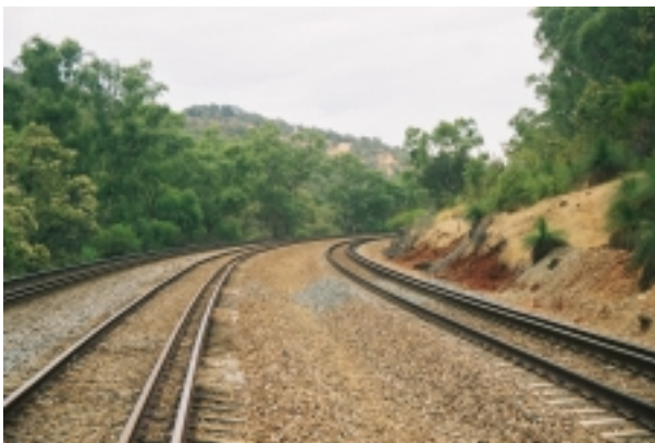
Figure 6 A location where off-train communication is difficult. The terrain will limit coverage to the rear of a train on this curve.
